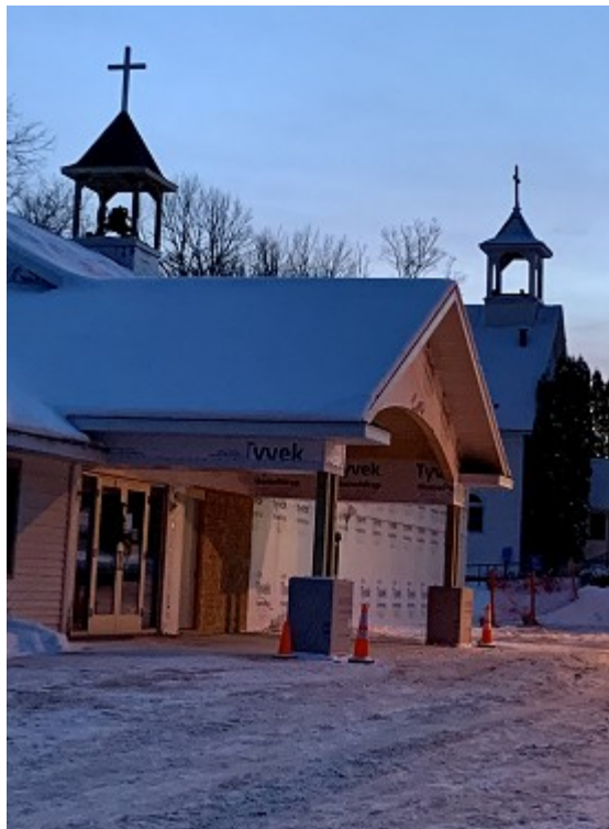
At the end of the day the old St. Anthony building begins to fade as the new building grows closer to completion.
